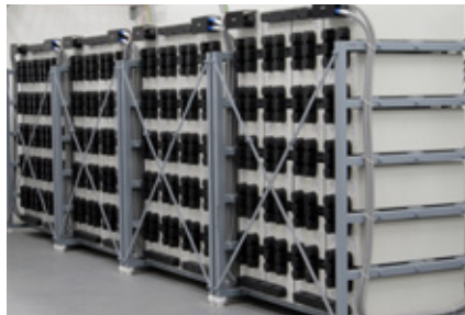
Energy Storage System
